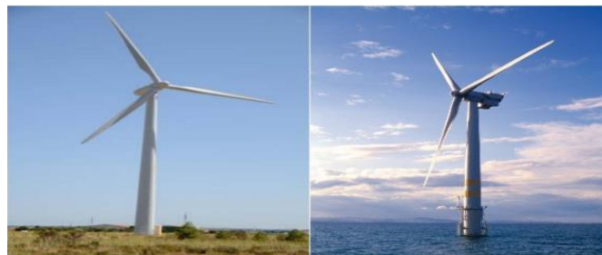
Figure 1.14. Horizontal- axis wind turbines [30].
