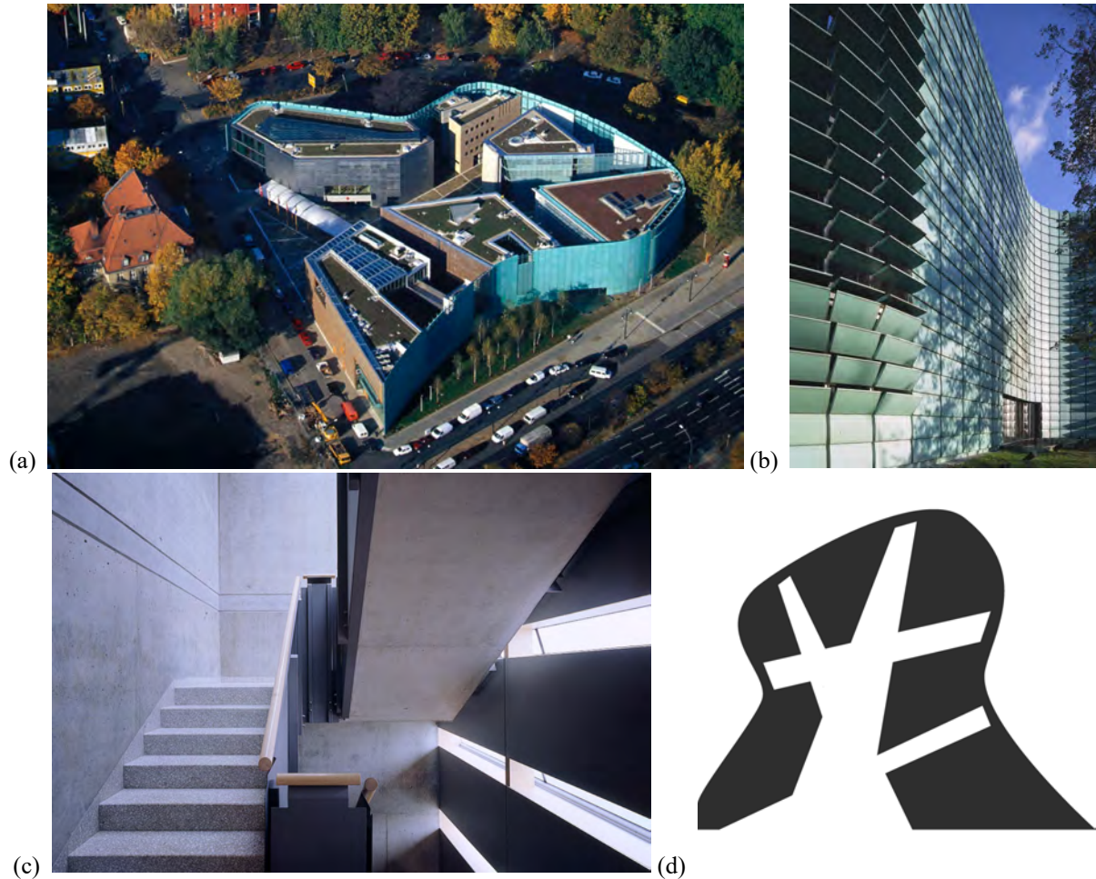
Figure 2-17. Berger + Parkkinen ( The Nordic Embassies, Germany 1995-99 ). Source: https://berger-parkkinen.com/en/nordic-embassies/ (Accessed date: November 27 th , 2021).
