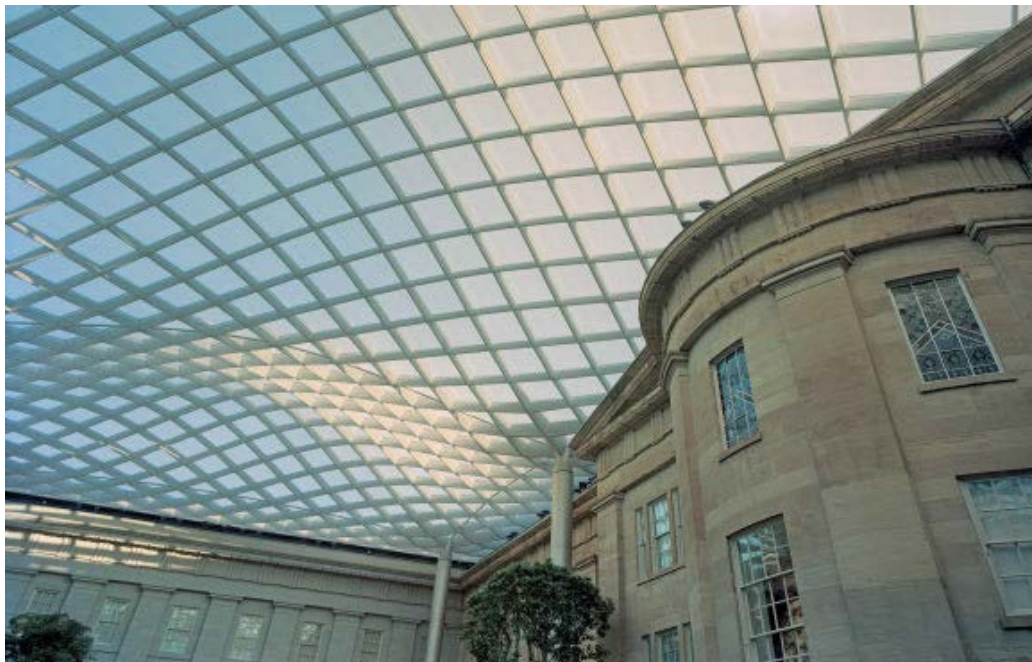
Figure 4-19. The Smithsonian's grid shell is built on a quadrangle system. (Mangelsdorf, 2010).
