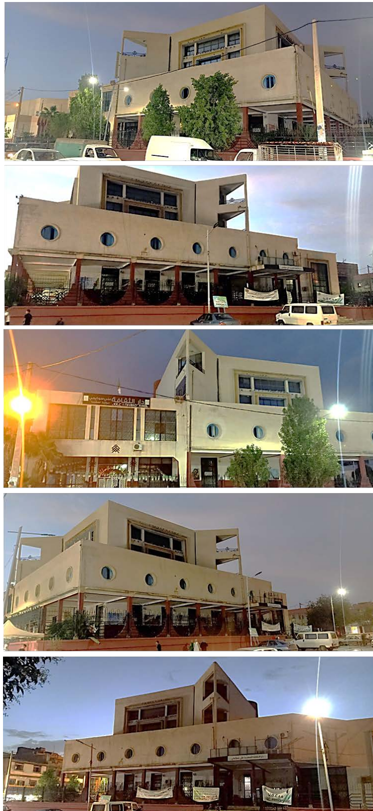
Figure 5-4. Views of the city of Khenchela's culture house (Source: Author, 2022).
