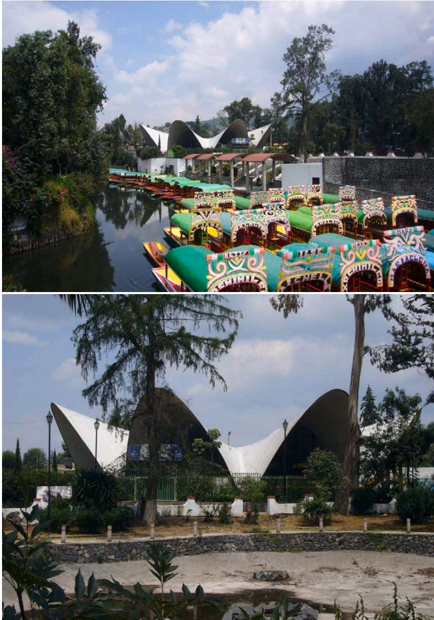
Figure 3-38. Restaurant Los Manantiales, Xochimilco, by Felix Candela (Source: Eugenio, E., & Parachini, M. (2011). Restaurante Los Manantiales / Félix Candela . www.archdaily.mx . Retrieved August 23, 2023, from https://www.archdaily.mx/mx/02-95859/clasicos-de-arquitectura-restaurante-los-manantiales-felix-candela .)
